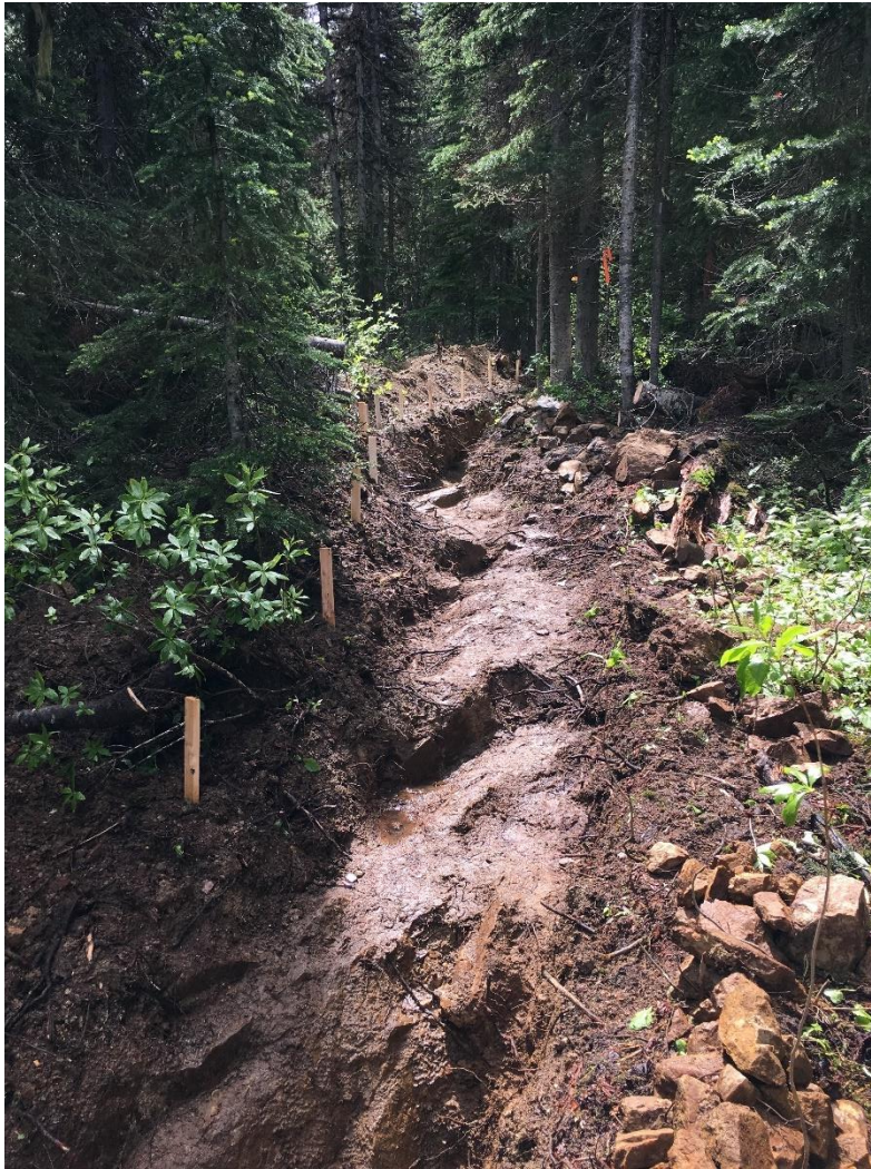
Figure 12. Picture of excavated trench at Twilight Zone, June 2019 (R. Ritchie, 2019).
