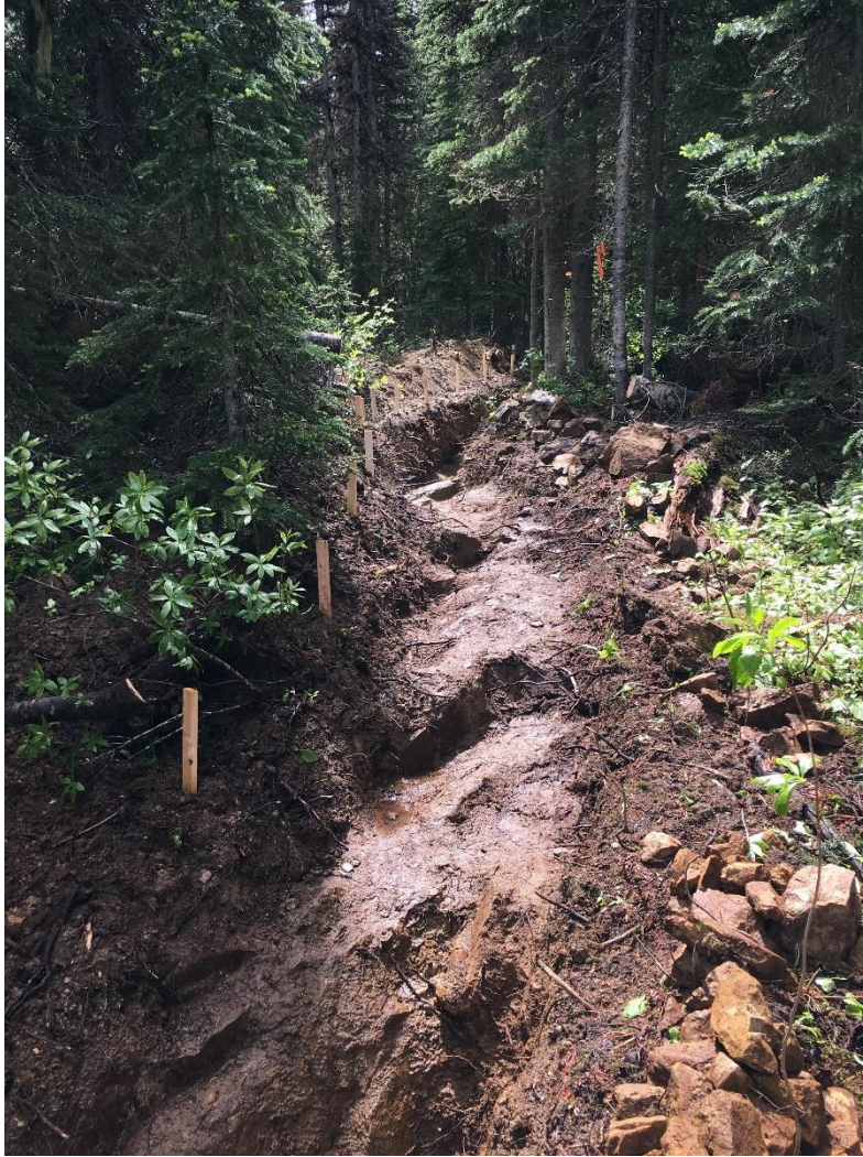
Figure 15. Picture of excavated trench at Twilight Zone, June 2019 (R. Ritchie, 2019).
