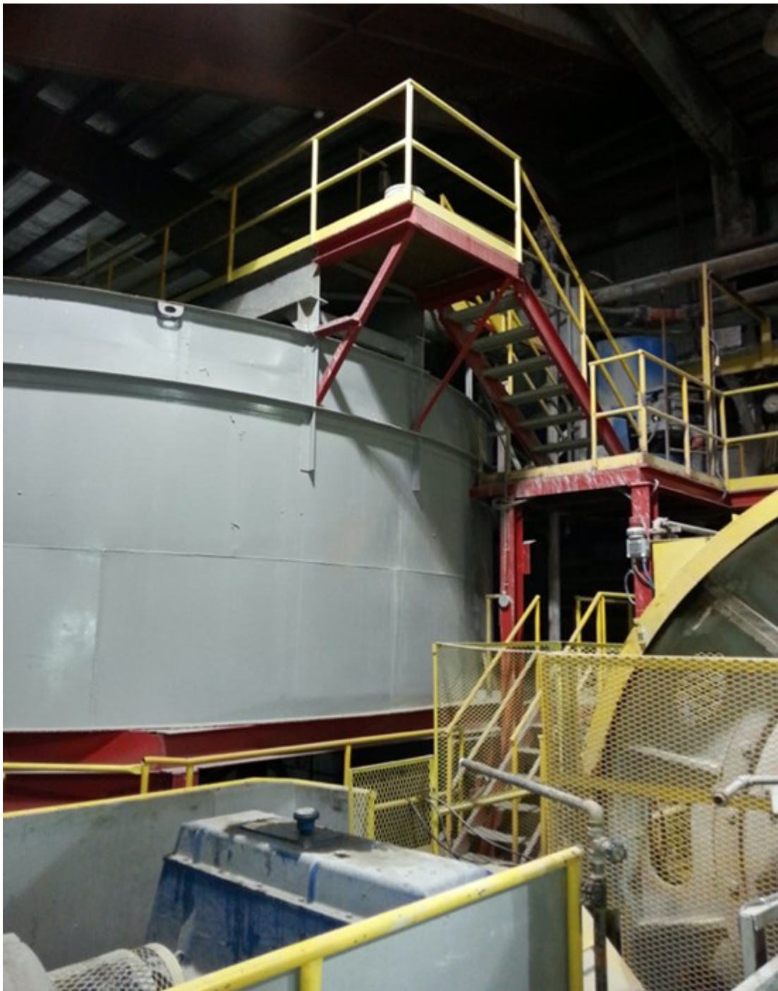
Figure 6: Photos of Beacon Mill and Property currently under care and maintenance
