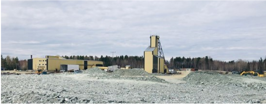
Figure 5: Photos of Beacon Mill and Property currently under care and maintenance
