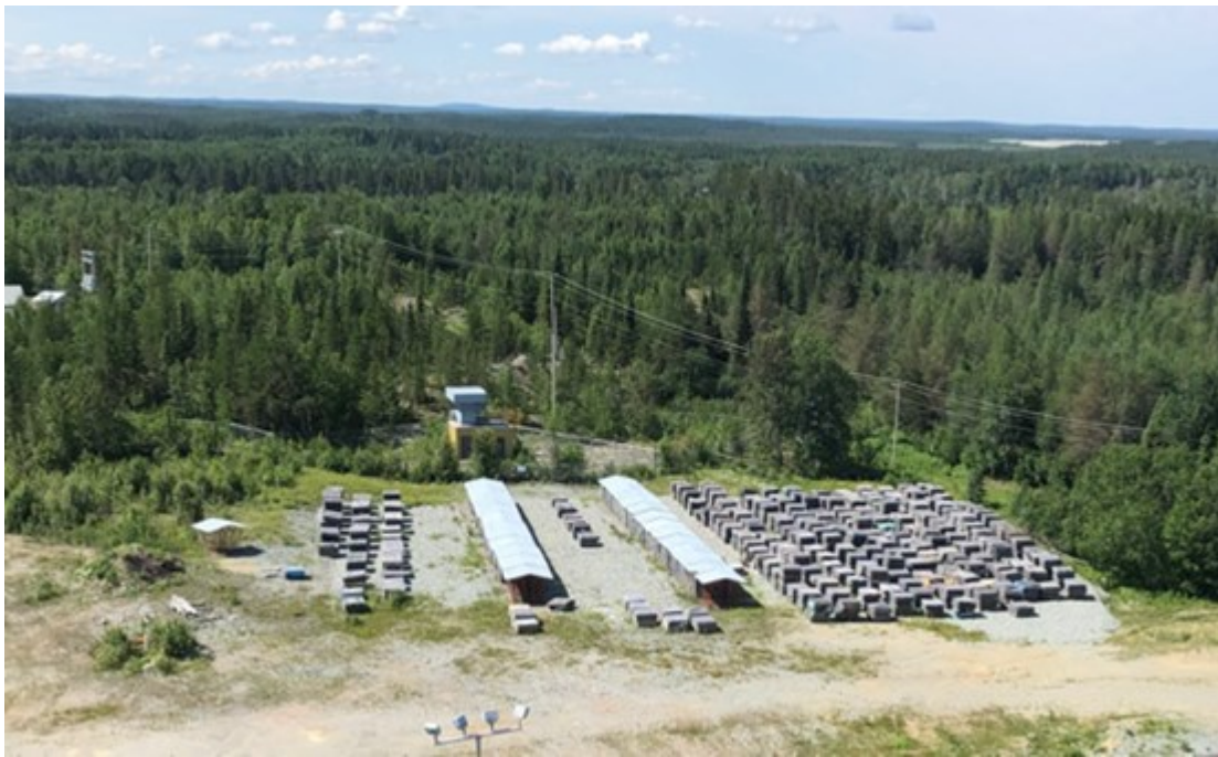
Figure 3: Photos of Beacon Mill and Property currently under care and maintenance
