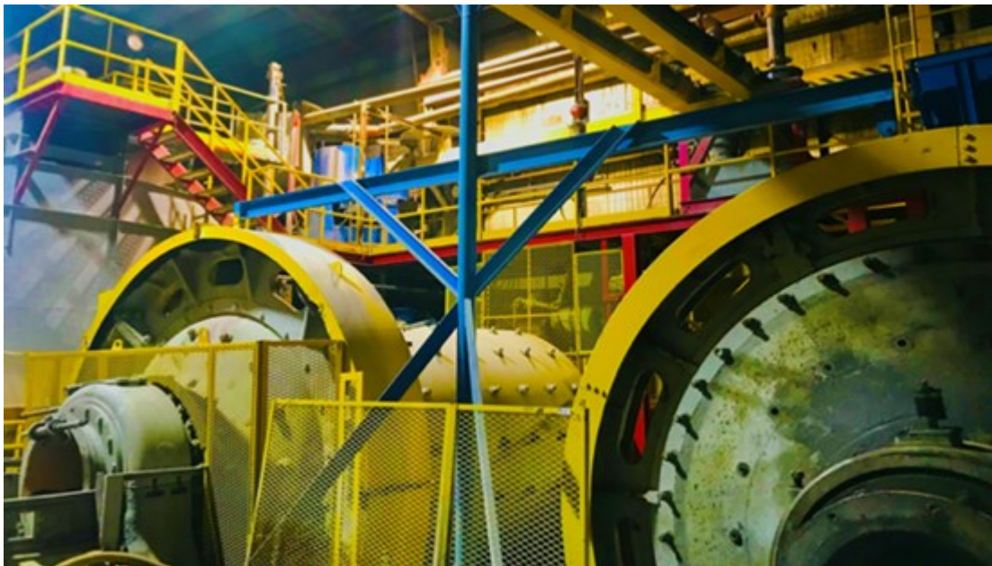
Figure 2: Photos of Beacon Mill and Property currently under care and maintenance
