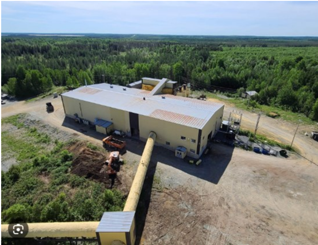
Figure 1: Photos of Beacon Mill and Property currently under care and maintenance
