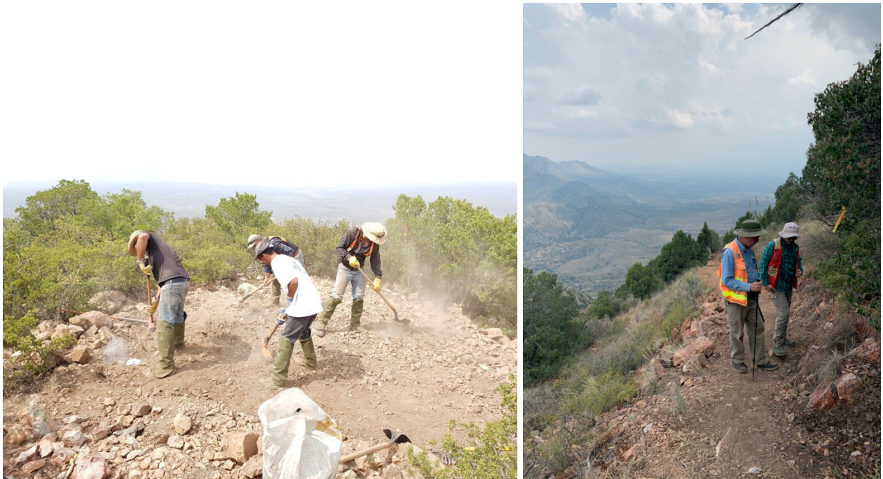
Figure 2: Drill pads being built and trails widened
