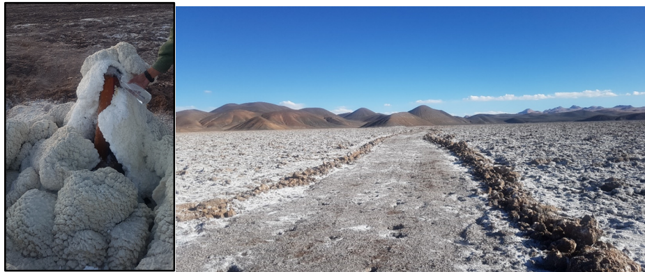
Figure 2 A Ganfeng drill hole which has brine coming up under salar pressure, and the access road to DDH 3,4 and 5.
