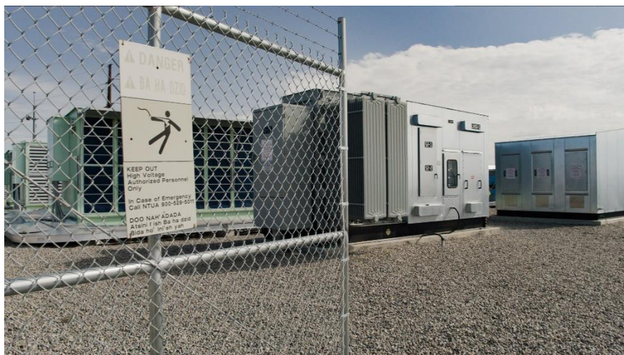
Entrance to LUXX Mining Operation in Shiprock, New Mexico.
