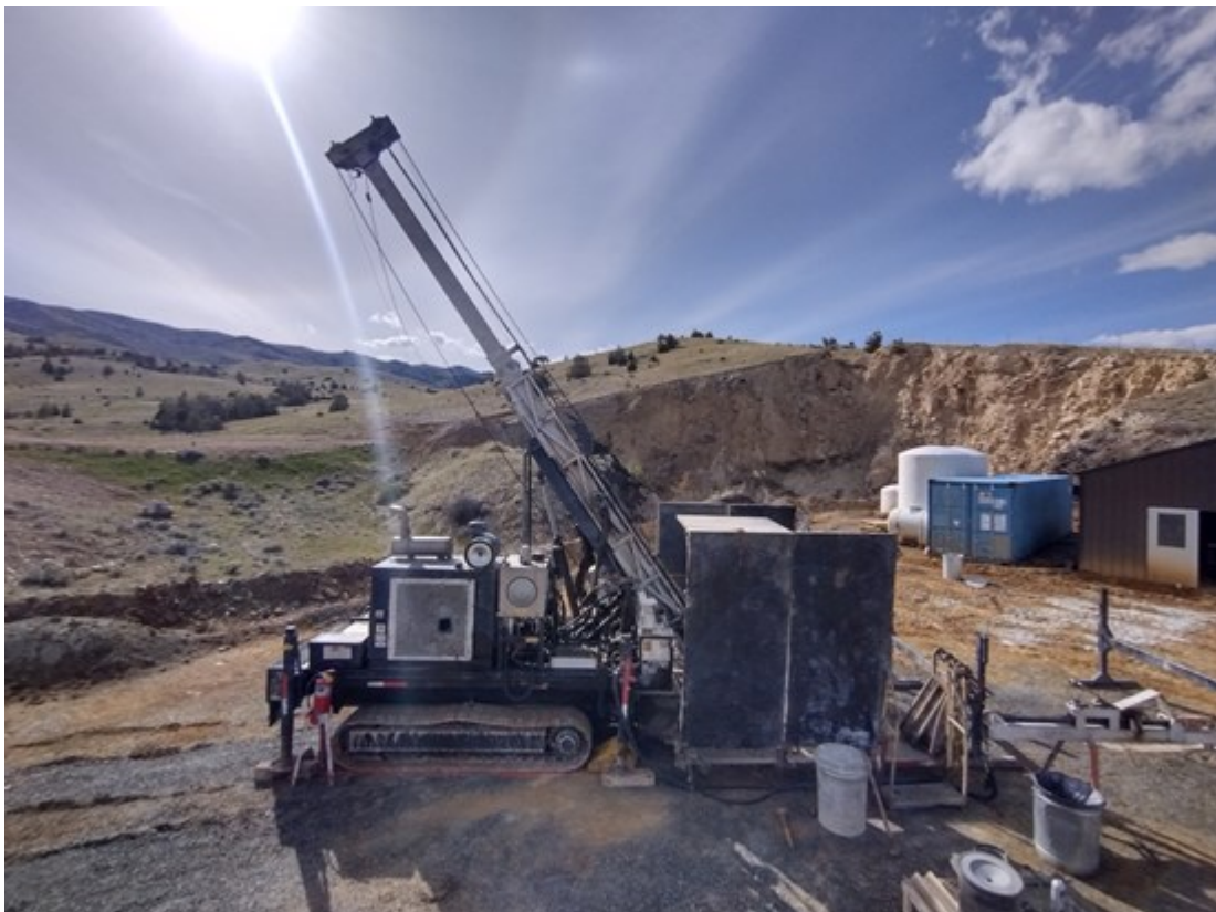
Figure 1. Drill rig set up in progress at Madison site
