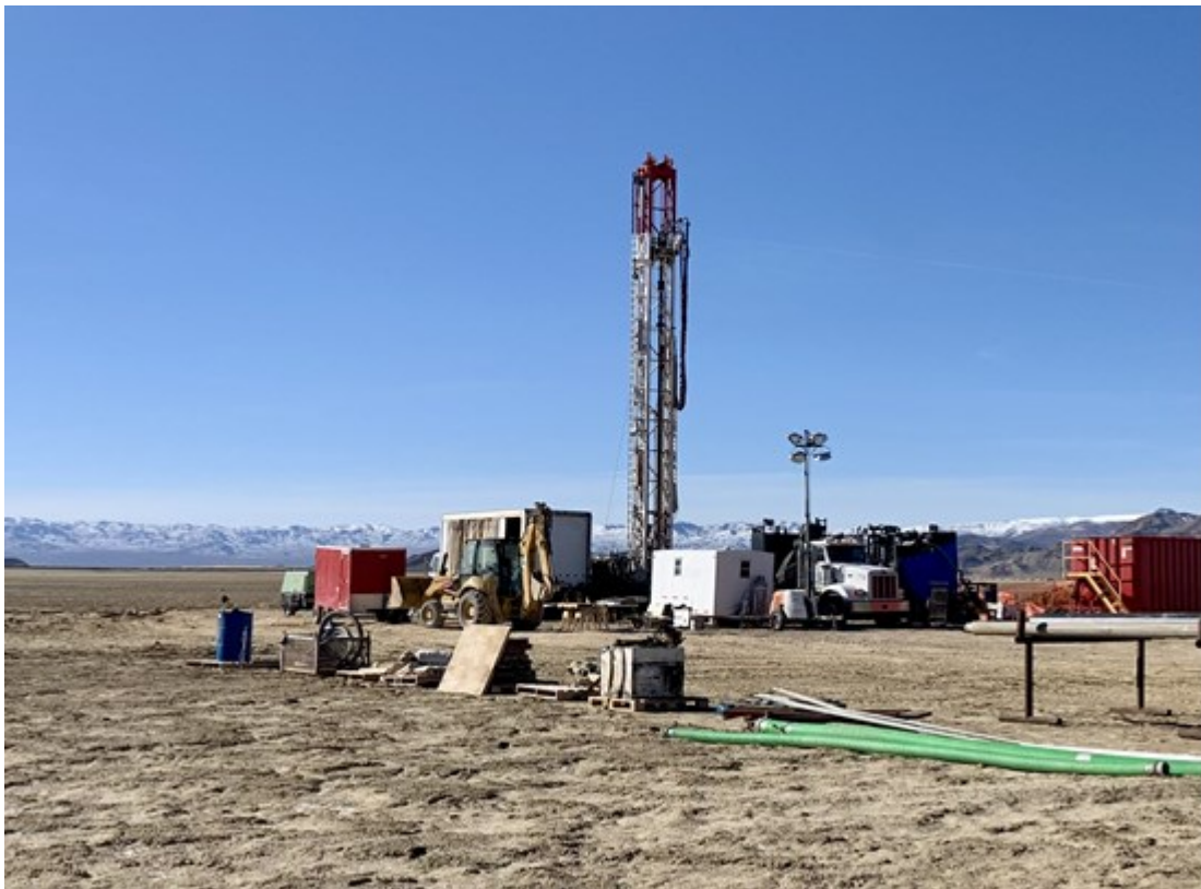
Drilling at Clayton Valley, Nevada (Fig. 1)
