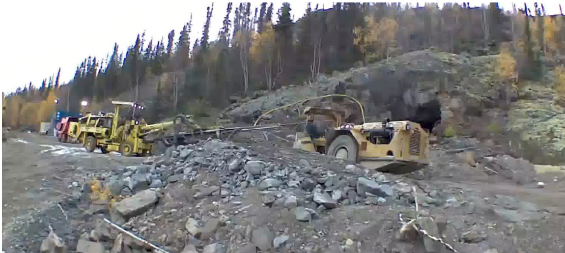
Photo 5. Electric hydraulic jumbo enroute to the ramp.
