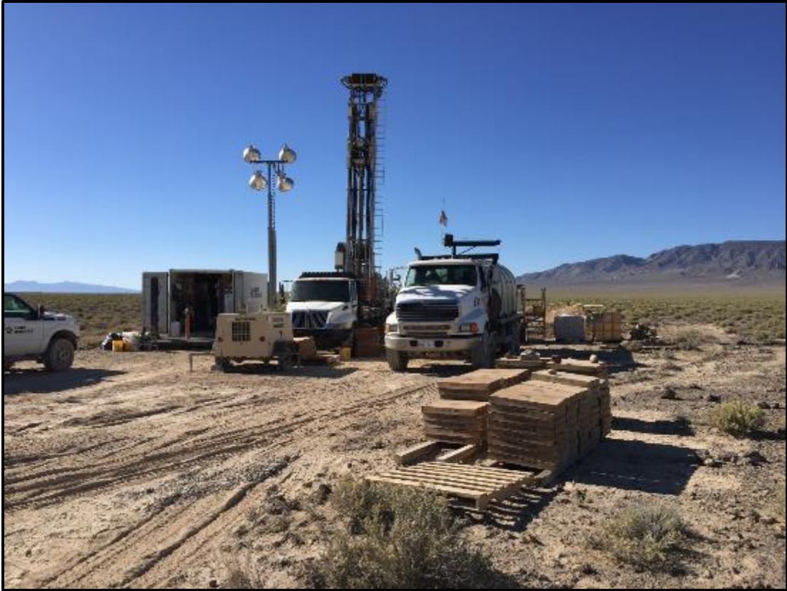
Photo 2: Drilling work in progress
