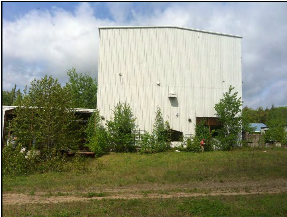
Photo 2: Historical graphite mill on the Property (Source: May 2015 property visit)
