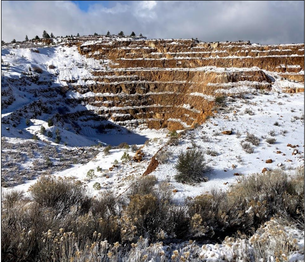
View of Lookout East Pit, Looking North (from Four Nines Gold Inc., 2022)
