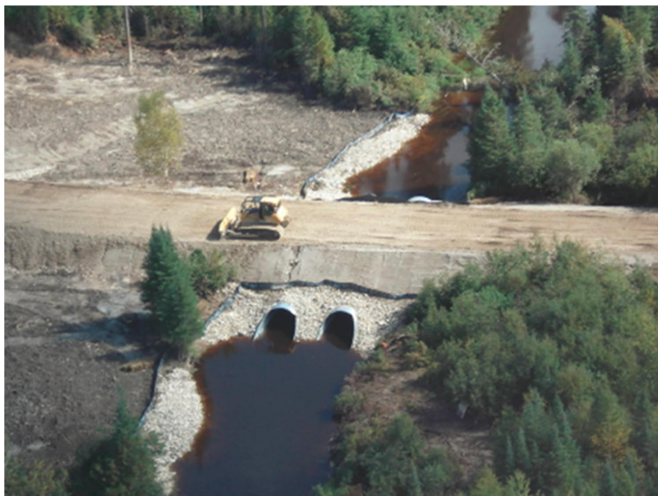
Figure 5-1: Fushimi Road – Fox River Culvert Construction
