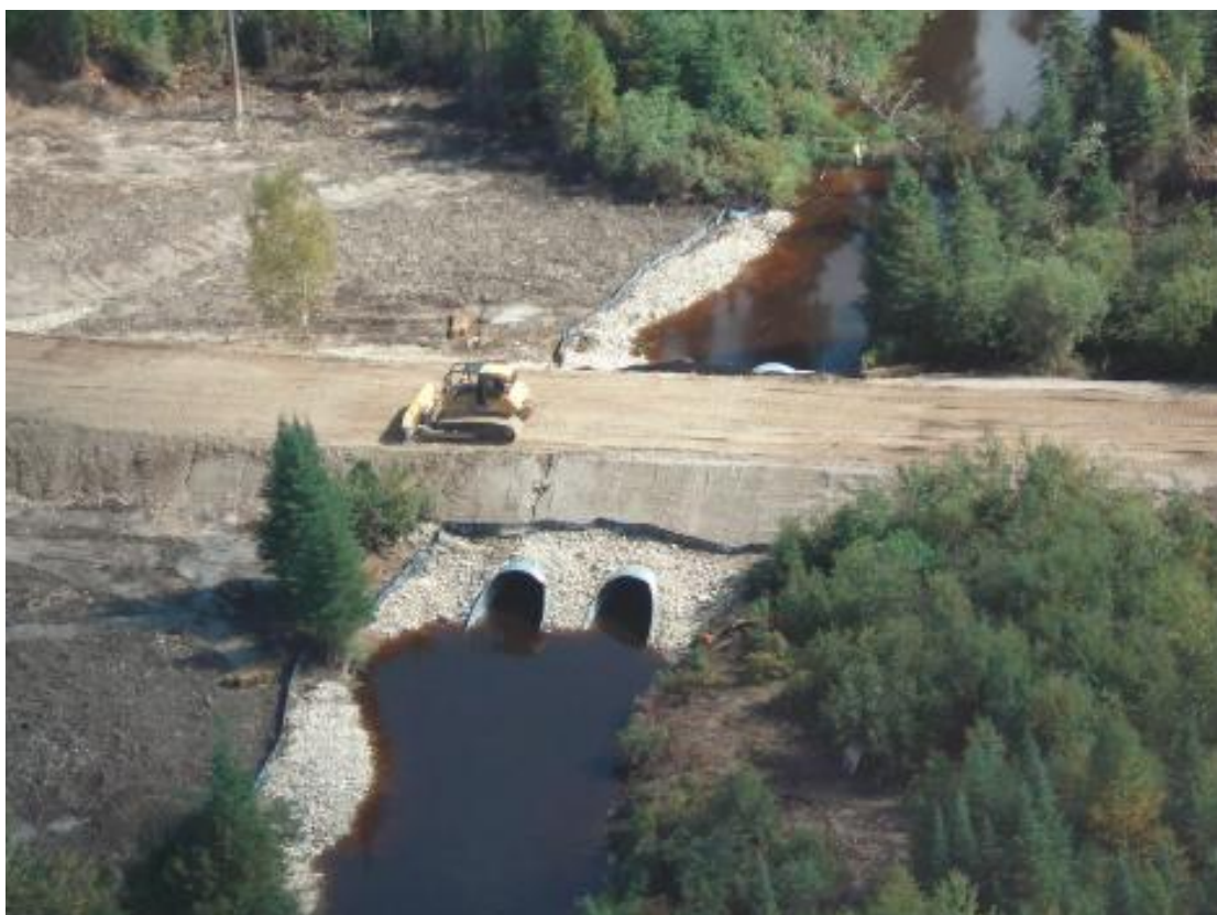
Figure 5-1 Fushimi Road - Fox River culvert construction
