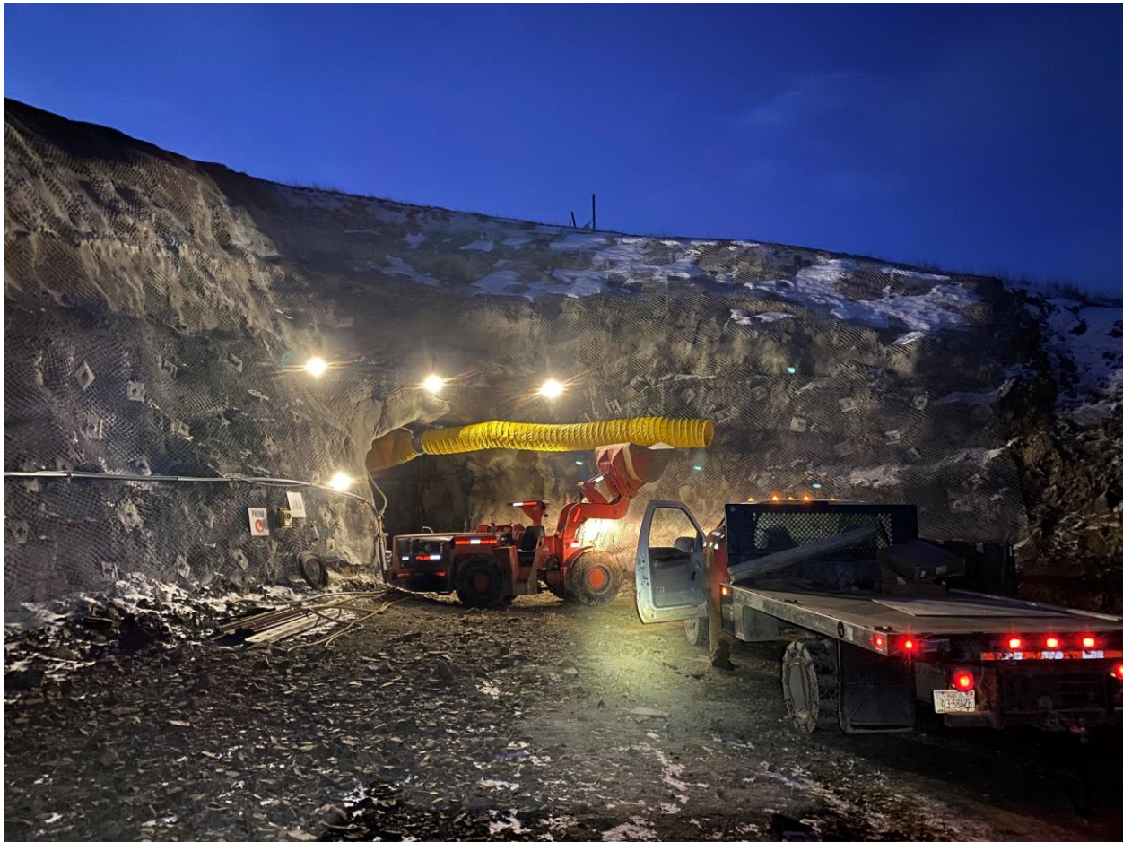
Image of Tunnel #1
