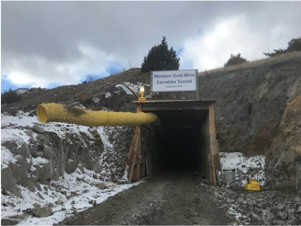
Images of Carrabba Tunnel Portal
