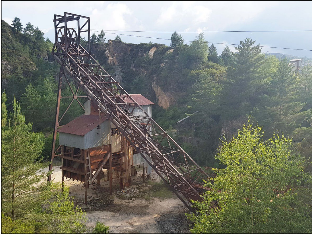
Photograph 4.2: Inclined Production Shaft in the Sta. Helena Breccia Open Pit
