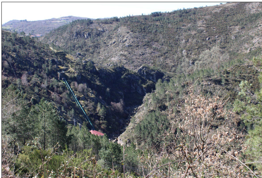
Photograph 4.3: View looking northward at the Borralha Penstocks and Power Plant
