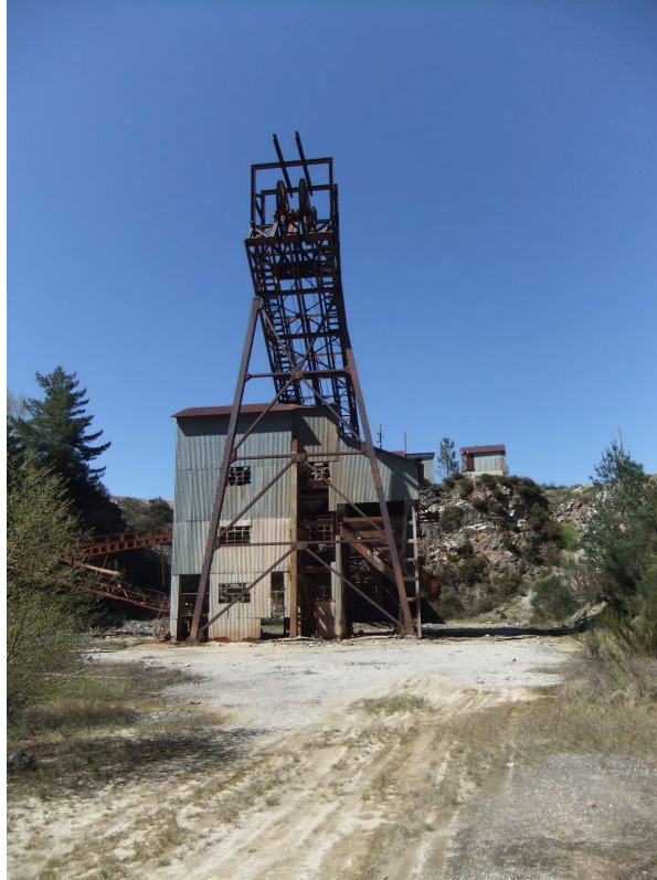
Photograph 9.1: Santa Helena shaft with Overgrown 2011 Trench 10 m to South (right)
