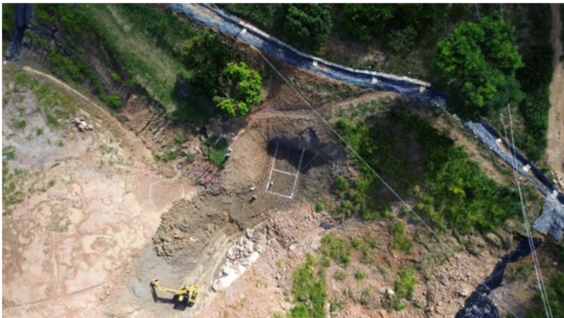
Figure 1 - Portal site construction commences November 12, 2024
