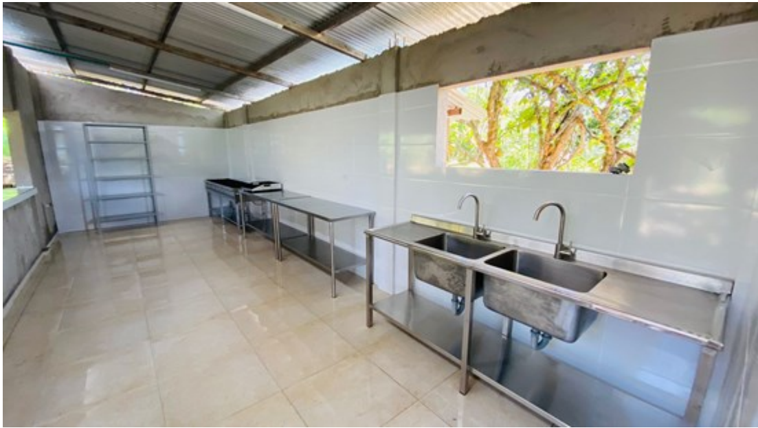
Figure # 4 - Camp kitchen construction nearing completion
