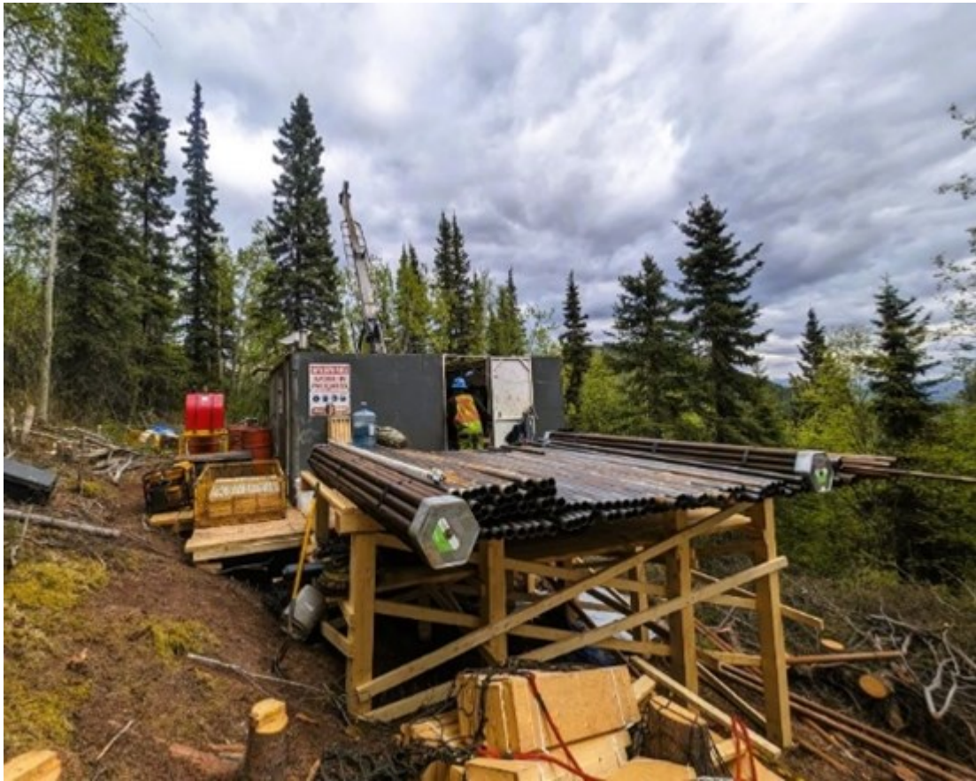
Figure 1 - ALT-24-001 Drill Platform
