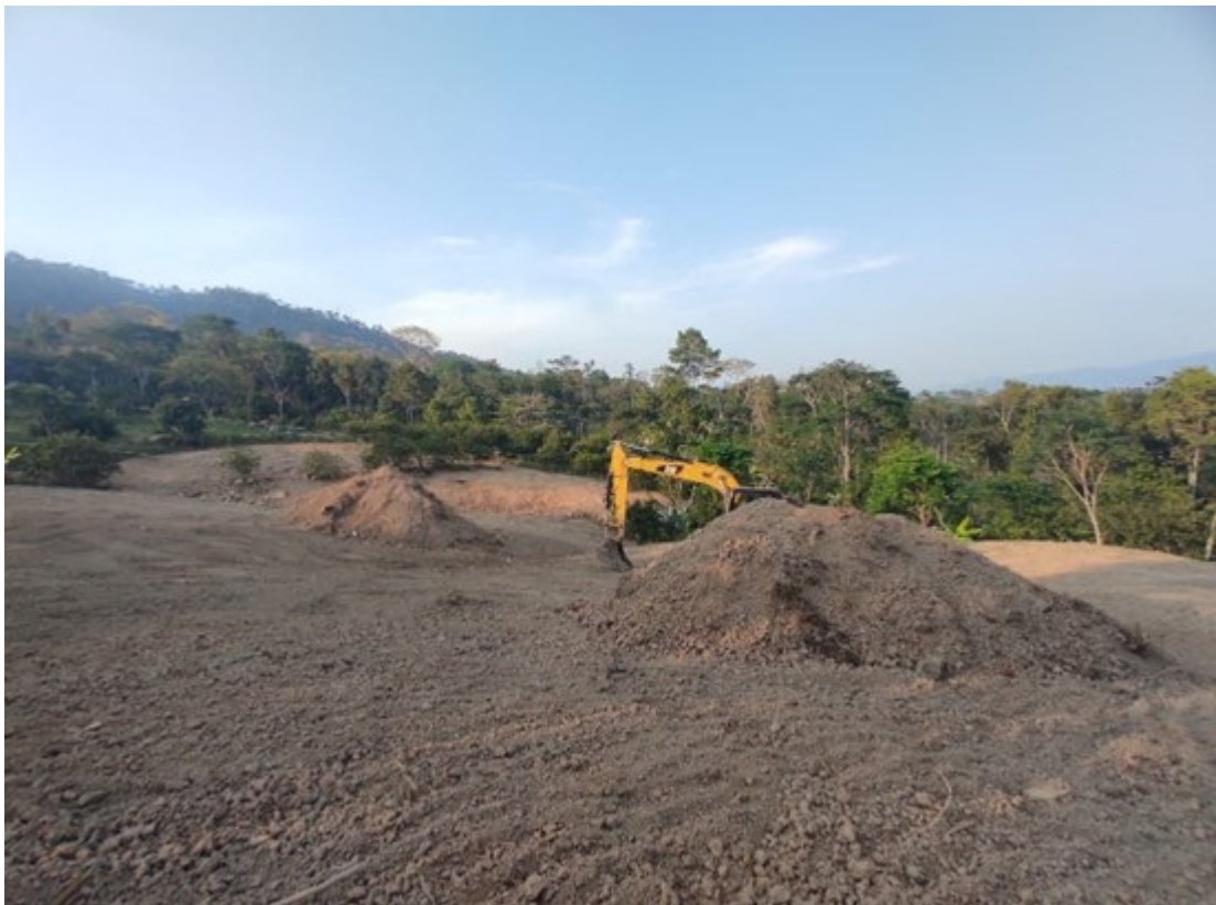
Figure 1. Surface preparation underway at La Estrella
