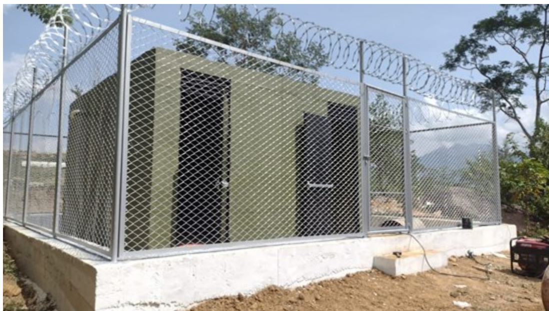
Figure 1 - Completed powder magazine
