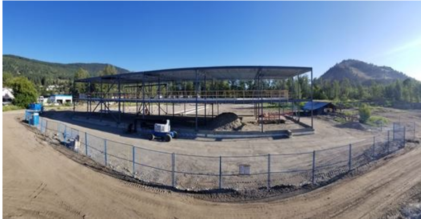
Figure 1: True Leaf's Campus Project construction as of July 2018
