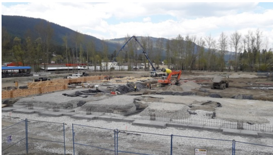
Construction of the True Leaf Campus Well Underway in Lumby, B.C.
