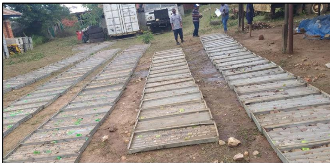
Figure 12-1. Core inspection during QP site visit.
