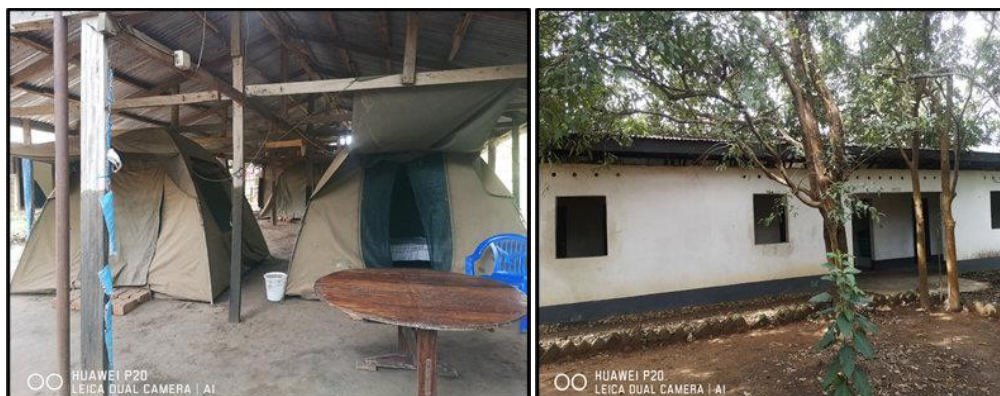
Figure 5-2. Camp site buildings observed during site visit, May 2021.
