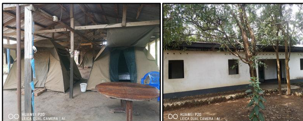
Figure 5-2. Camp site buildings observed during site visit, May 2021.
