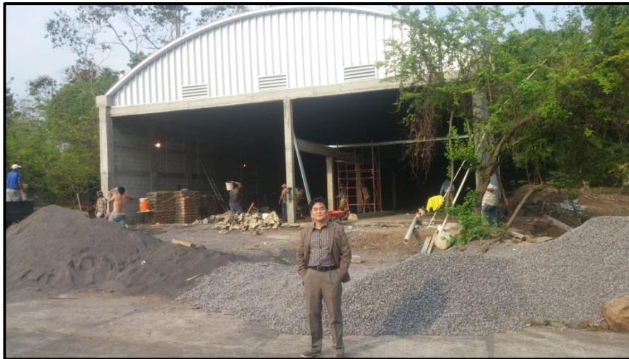
The Company's CFO, James Choi at the Guatemala Factory during construction.
