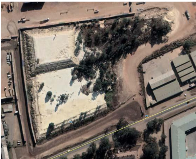
Figure 1 Aerial photo of the tailings site
