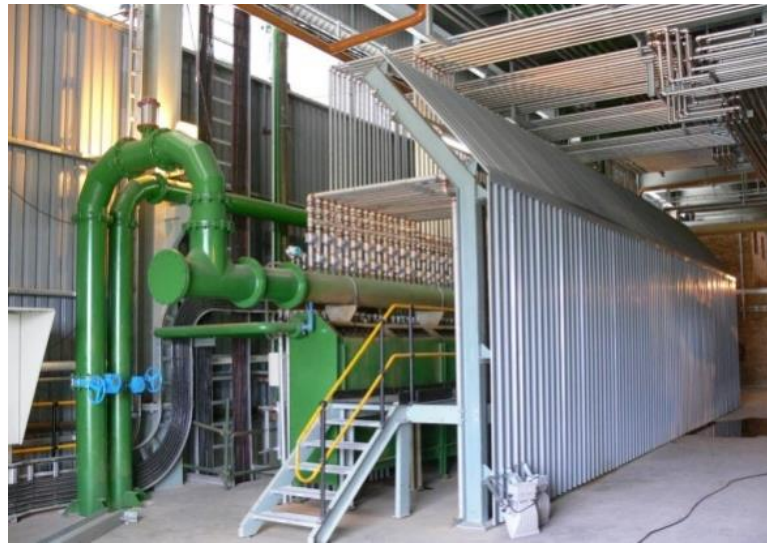
Figure 104: SAF cooling water system
