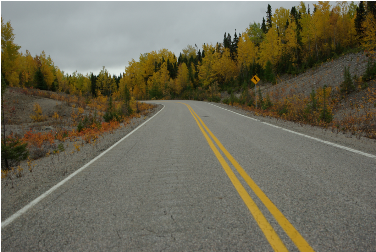
General view of the Selbaie road used to access the property
