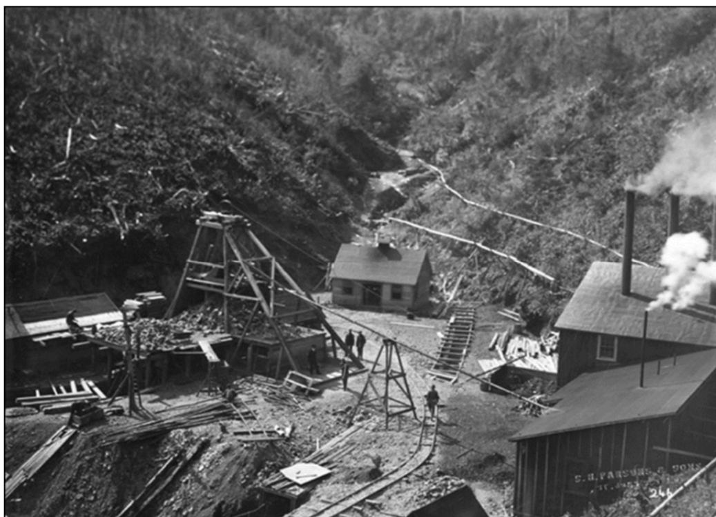
Figure 6-1: York Harbour “A” Zone Shaft and Mine Buildings (ca. 1899-1913)
