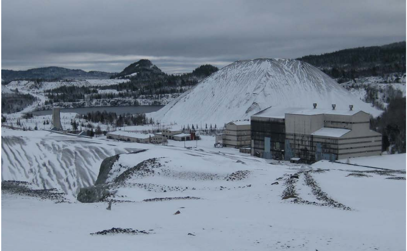
Figure 6.1: View of Normandie mine infrastructure looking SE from top of Tailings. Normandie open pit (water-filled) in background behind Penhale headframe. Normandie secondary tailings pile behind main mill building.
