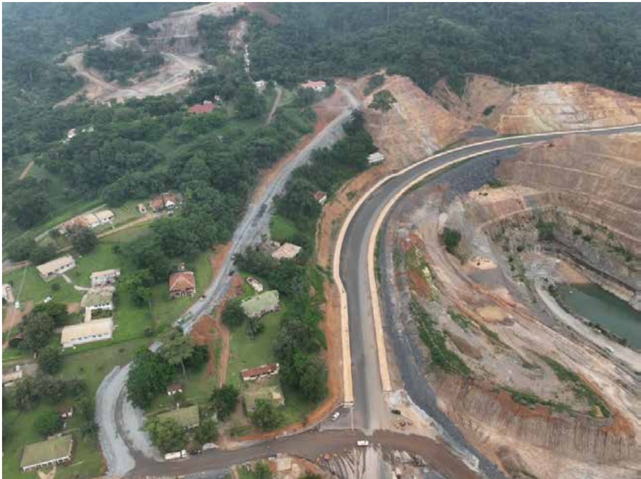
Figure 1 – New road alongside Bibiani Pit
