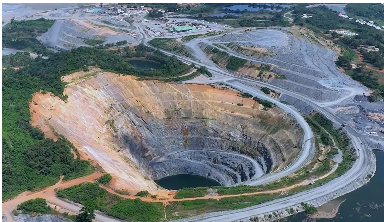
Figure 7-14: Drone Picture of Walsh Pit Looking North (Source: MultiGeomatics; Land Mining & Engineering Surveyors 2023)
