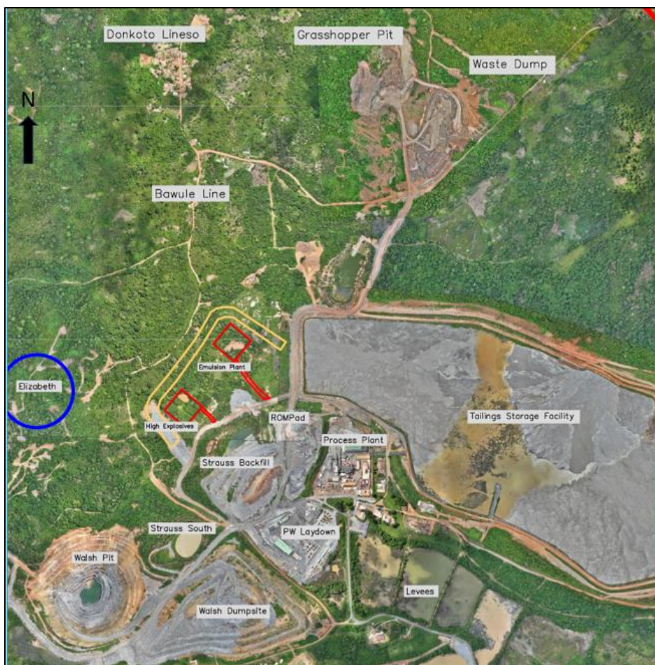
Figure 5-2: Bibiani Gold Mine – Open Pits and Surface Infrastructure
