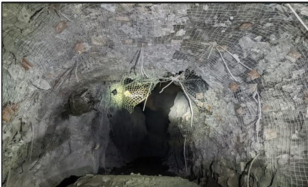
Figure 16-10: Akwaaba 1575 Ore Drive
