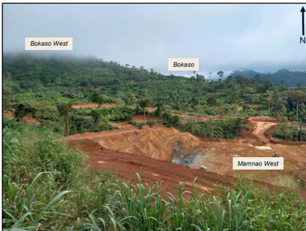
Figure 10-13: Mamnao Open Pit looking North towards Bibiani Mine
