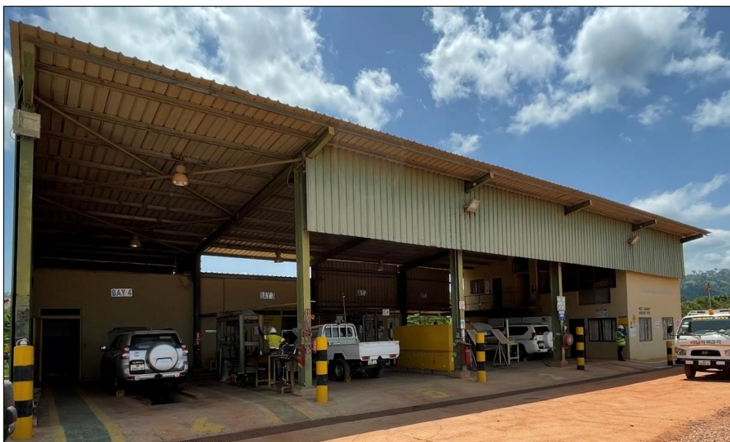
Figure 18-5: Light Vehicle Workshop
