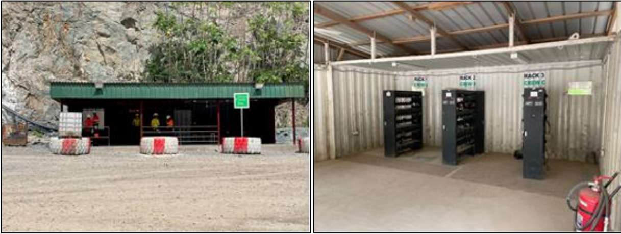
Figure 18-15: Security Control and Lamp Room Facilities at the Portals
