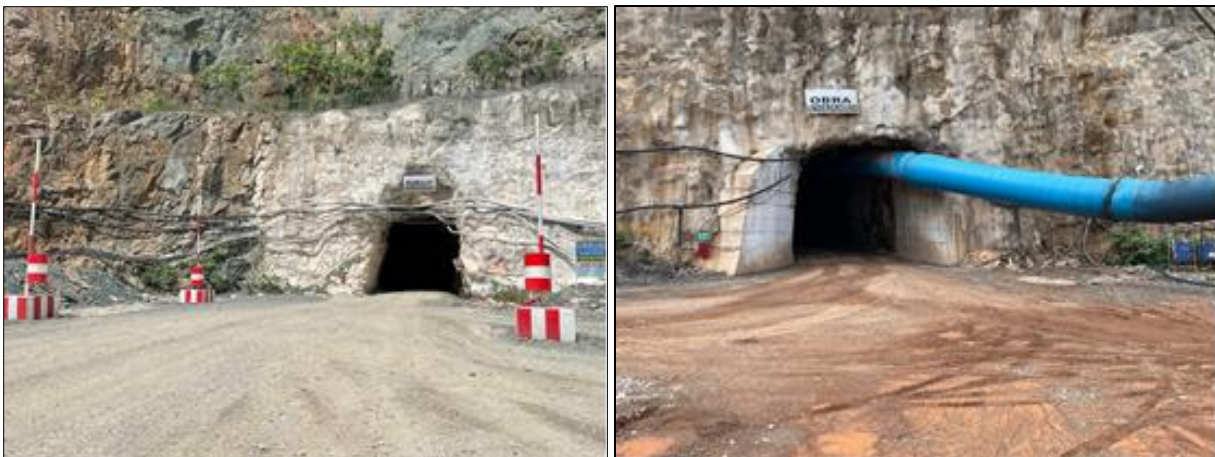
Figure 18-14: Suraw and Obra Portals
