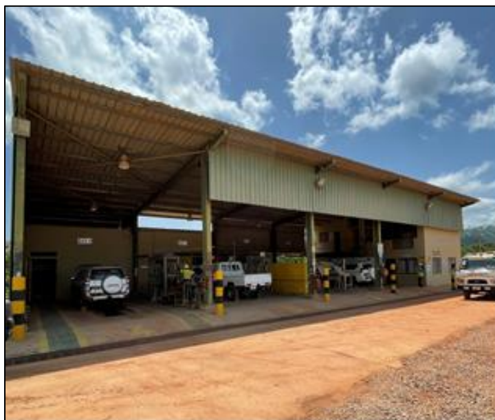
Figure 18-6: Light Vehicle Workshop
