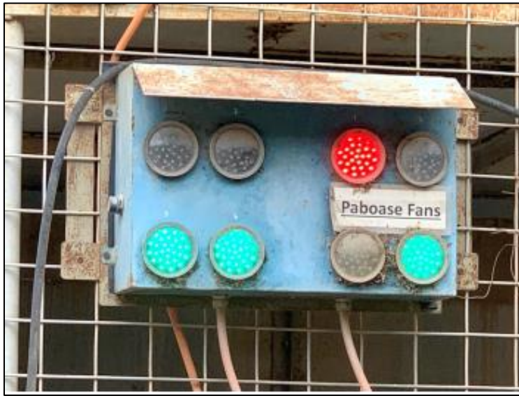
Figure 18-21: Primary Fans Indicator Lights
