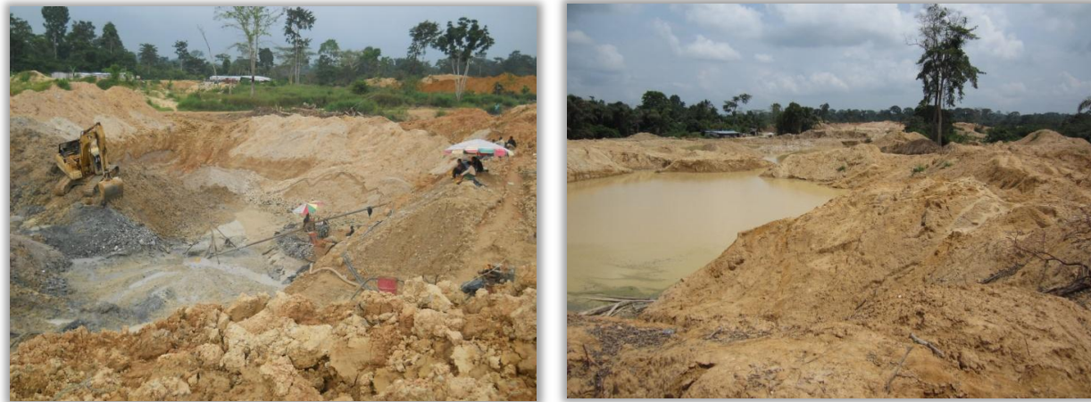
Figure 5.4.2 Typical galamsey alluvial operations in concession area
