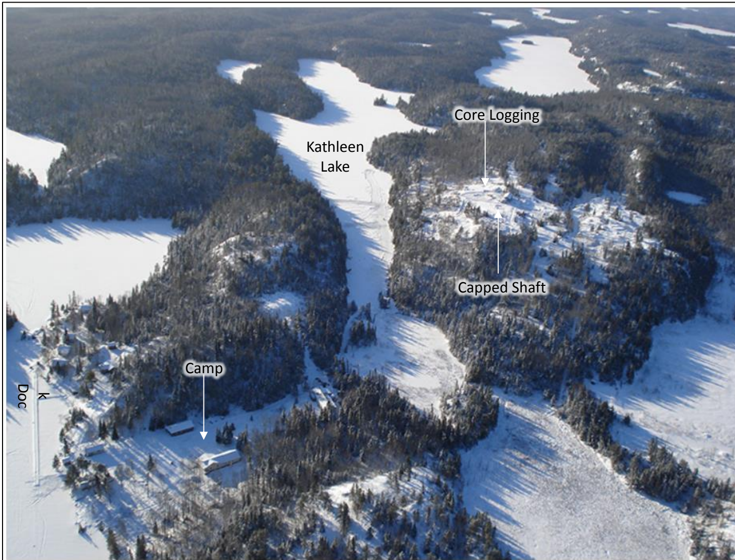
FIGURE 18.1 AERIAL VIEW OF INFRASTRUCTURE ON THE KENBRIDGE PROPERTY NEAR KATHLEEN LAKE
