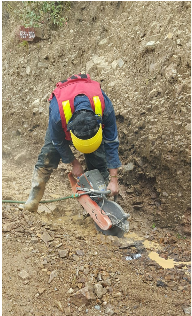
Figure 11.1. Picture of a worker cutting rock with a gasoline-powered diamond blade saw.
