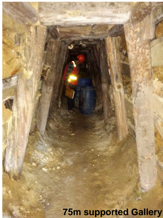
Figure 7.12. Picture of a Timber-supported gallery within the Rufina zone.
