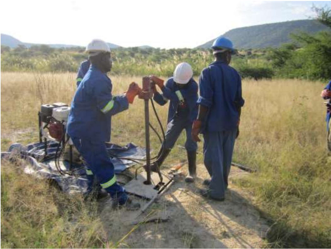
Figure 10-1 Power auger drilling
