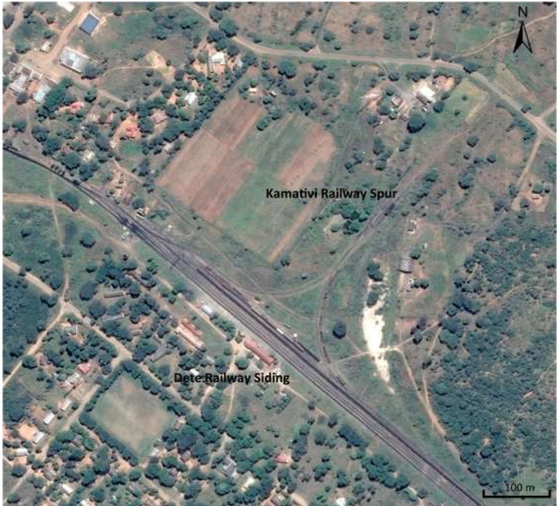
Figure 5-5 Aerial image of the Dete railway siding
