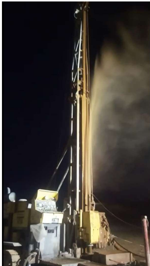
Figure 6-4 Picture of the brine surge from DDH2 at approximately 407m depth
