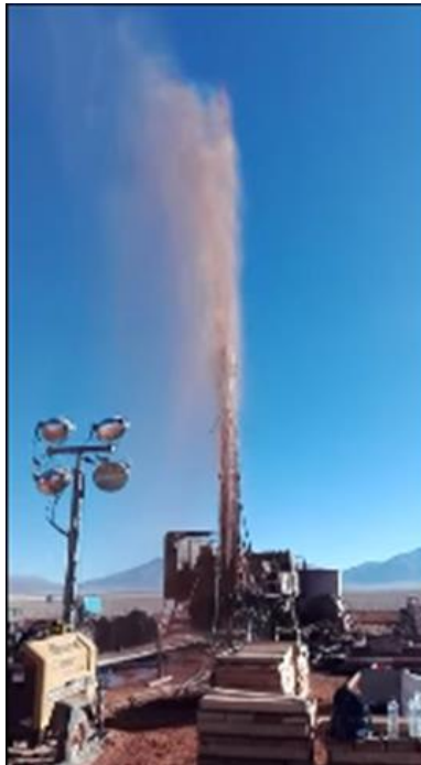
Fig 3. 2018 Drilling at Pocitos 1
