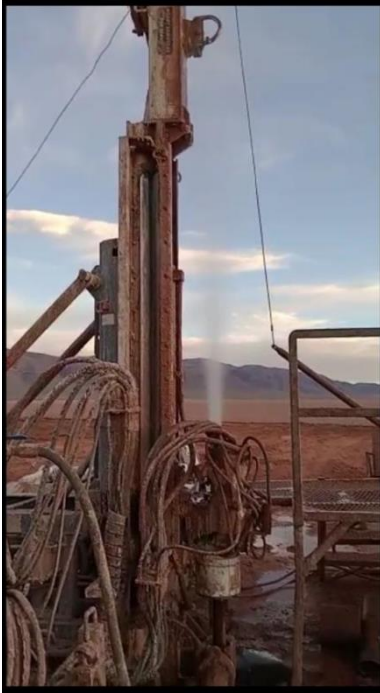
Fig 2. Dec, 2022 Drilling at Pocitos 1
