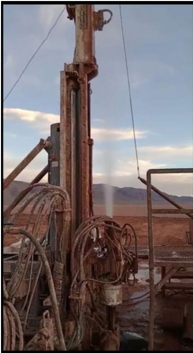
Fig 1. Dec, 2022 Drilling at Pocitos 1
