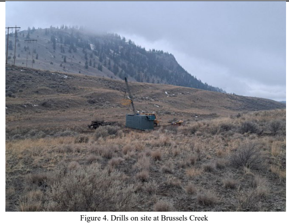
Figure 4. Drills on site at Brussels Creek
