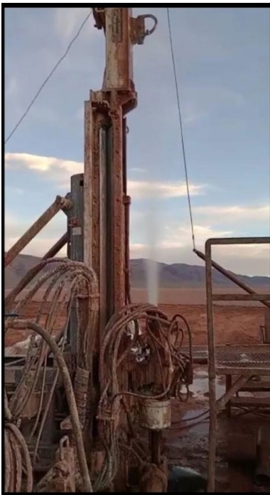
Fig 1. Dec, 2022 Drilling at Pocitos 1
