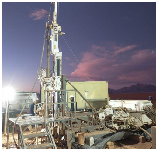
Figure 2. Drilling commences at Pocitos 1
