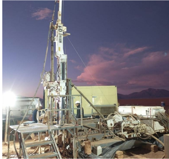
Figure 2. Drilling commences at Pocitos 1
