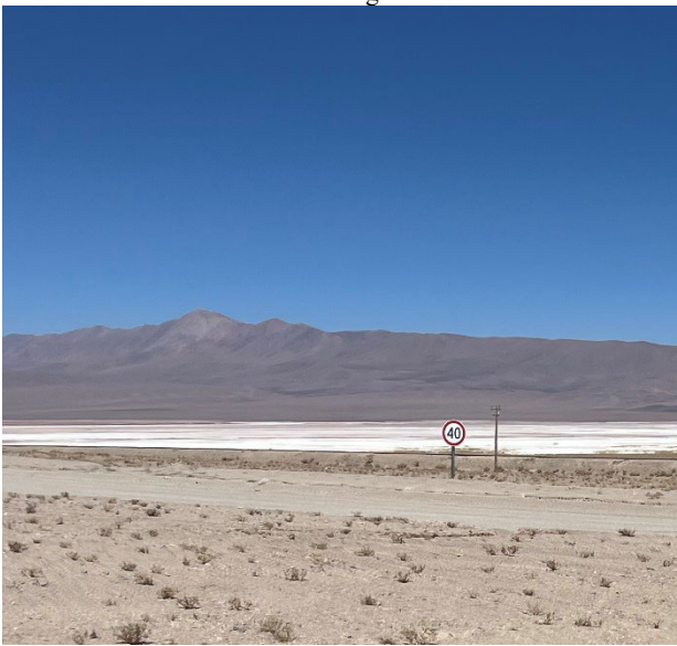
Figure 3. Pocitos Salar with gas, power and rail to Antofagasta, Chile Port
