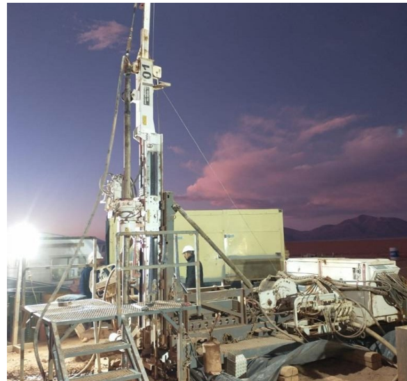
Figure 2. Drilling commences at Pocitos 1
