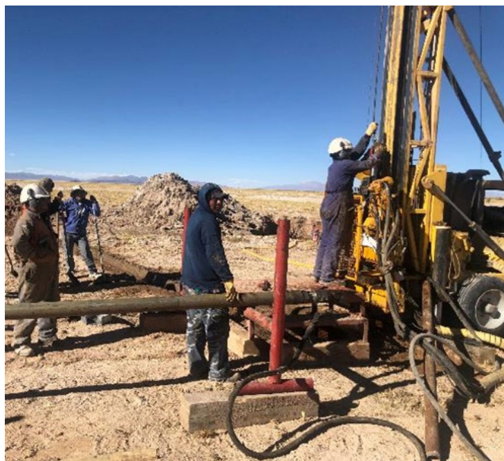
Figure 1. Drill on site from 2018 drilling campaign
